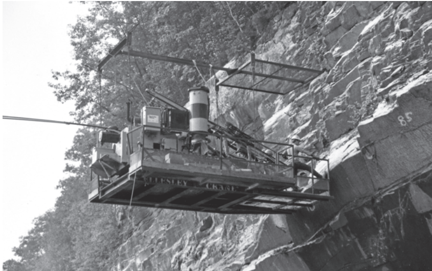
Platform rock bolting in the early 1990s.
