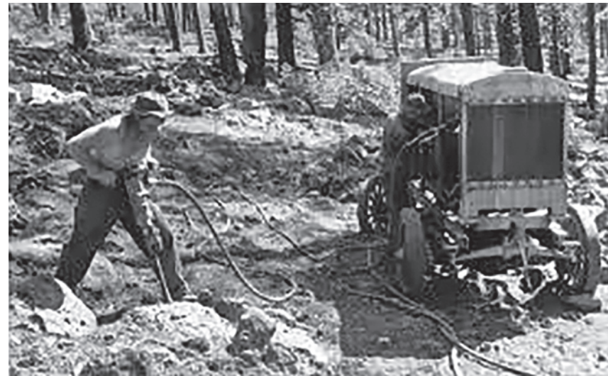
A jackhammer with the Sullair compressor and long hose. Much of the drilling was done this way in the early days.
