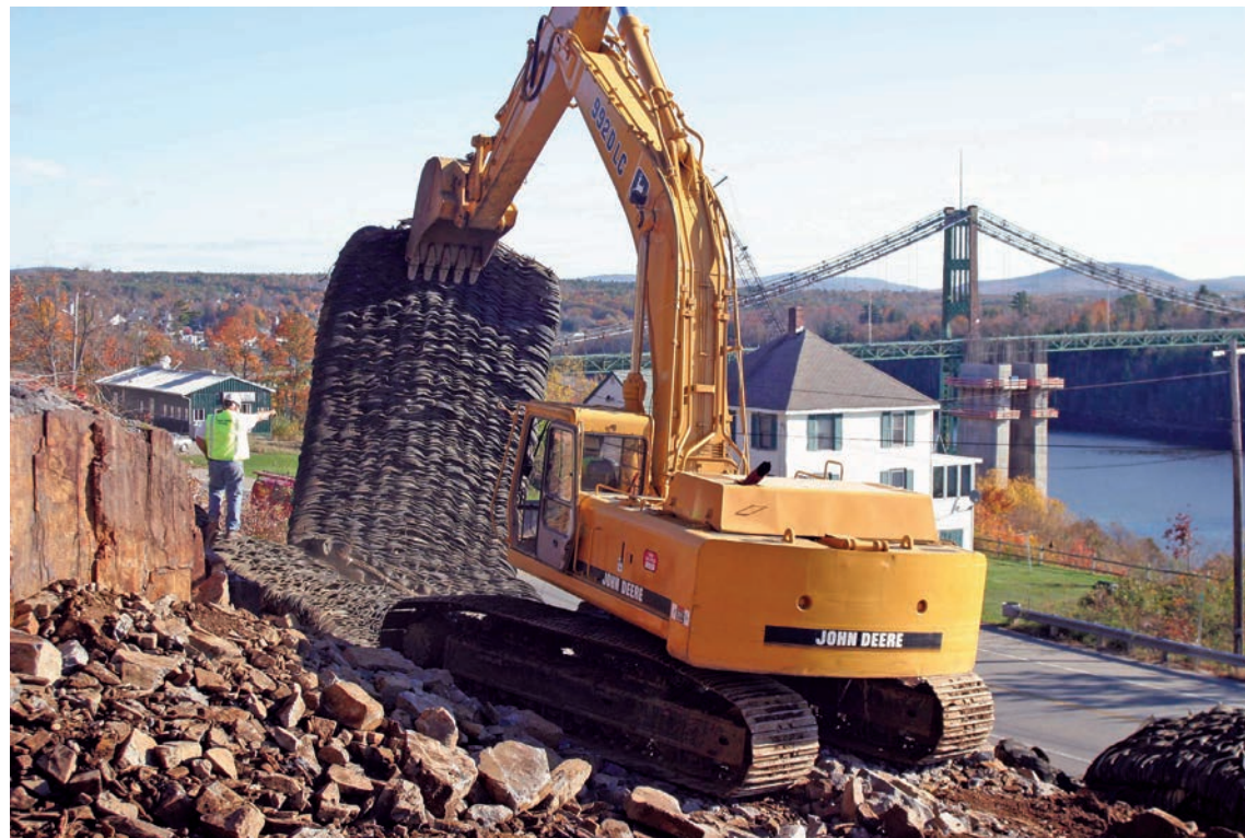
Laying the blasting mats along the Penobscot River.
