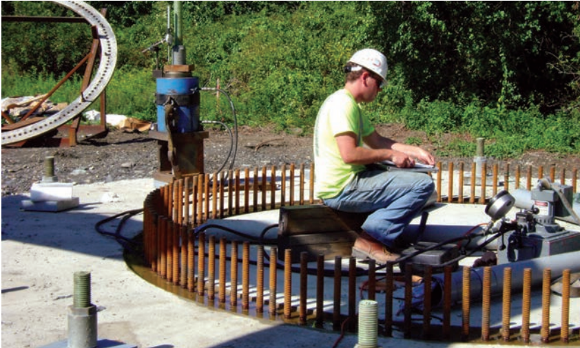
Peter Marcotte testing rock bolts on windmill pad.
