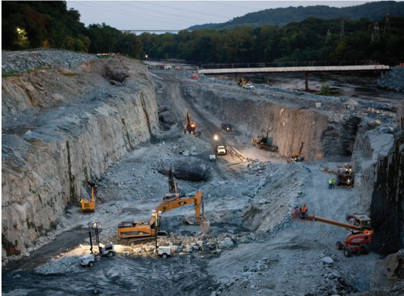
Operations went uninterrupted as days turned into nights at the Holtwood Hydroelectric Plant expansion in Holtwood, Pennsylvania. Drilling, excavation, and rock anchor installation all worked together in the ever-deepening footprint of the new powerhouse.
