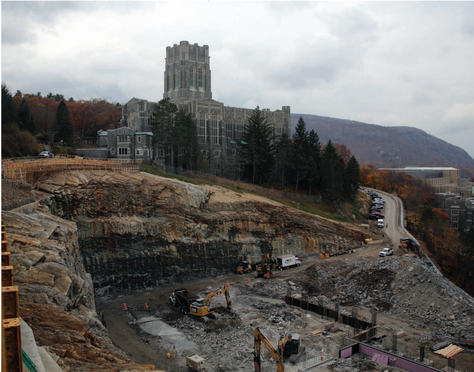
The West Point pre-split and retaining wall, with the chapel in the background.
