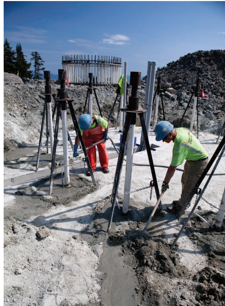
Eric Gallagher (in orange); Ben Kramer on right rock bolting the pad.
