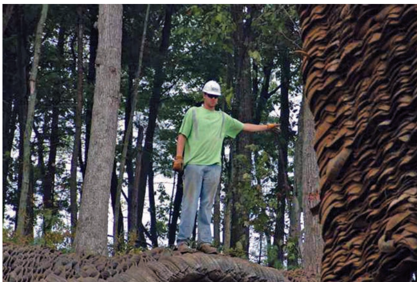
Dan Werner directing the setting of blasting mats.
