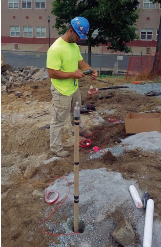
Construction Superintendent Trainee, John Jagger, training in Digi-shot electronic detonation systems, Malden, Massachusetts.
