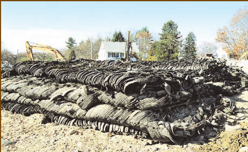
Extra heavy rubber-tire blankets are used to muffle shots.
