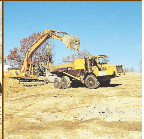
Hyundai excavator loads blasted rock fragments into Cat 250D off-highway hauler.
