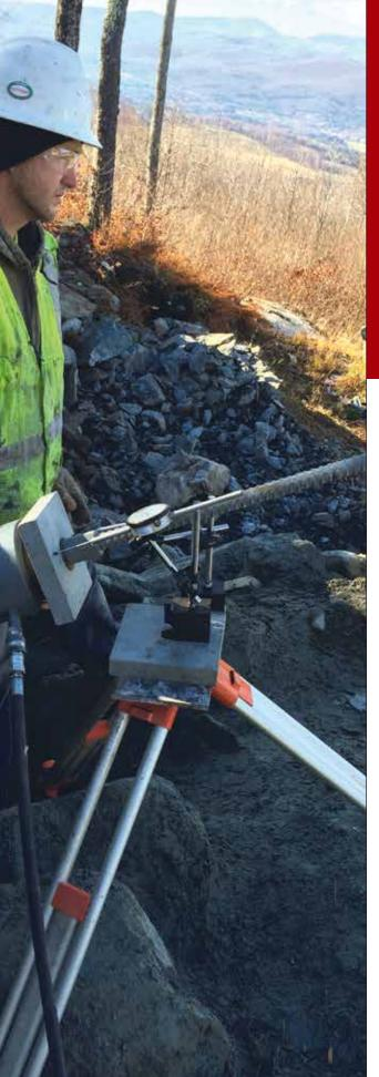
Early morning load testing of 20 kip rock anchors to stabilize a rock face above a patio/pool. MD&B recessed the bearing plate assemblies so that the anchors could be blended into the rock face with a color matched grout pack. Private Residence, Stowe Vermont. MD&B Blaster, Dean Butler.
