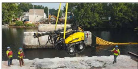
Utilizing a tight-access, light-weight T-15 to drill for rock dowels on the Biddeford Bridge Project, Maine
