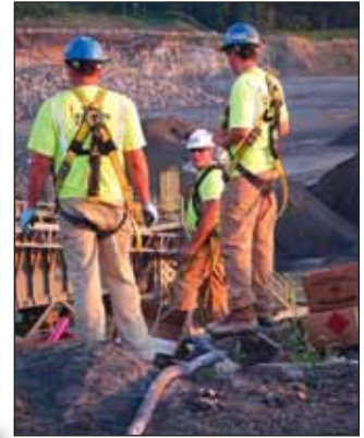
Blaster in charge Todd Larain, center, giving instructions to the crew.
