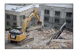
**Scope:** Controlled blasting for 135,000 yards of mass rock and 60,000 sqft of line drilling/presplit to make way for the construction of a new Cadet Barracks at West Point Military Academy Campus, New York.
