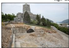
ensure the position and quality of our drilled holes prior to the loading. It took a team effort with all the trades/GC to orchestrate the 175+ blasts. Each one involved operating over 15 seismographs to be maintained and 14 personnel for site security before each blast was initiated.
